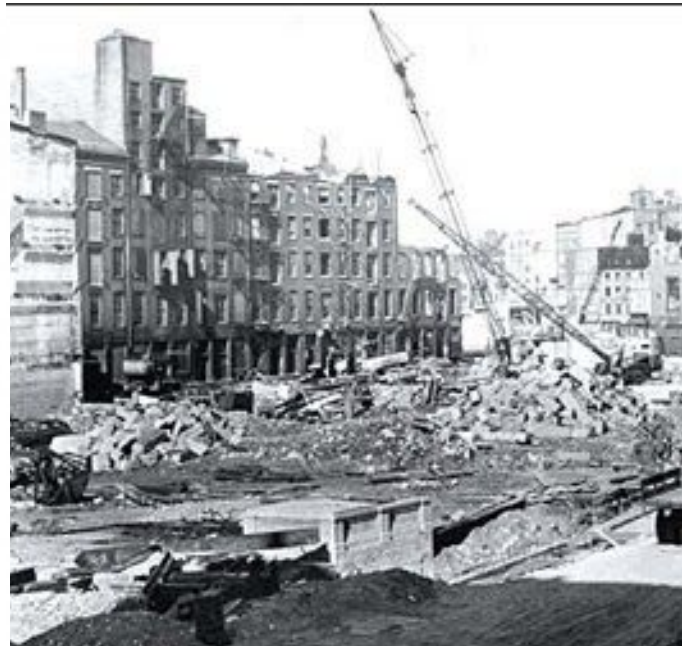
D. Picture of Urban Decay
